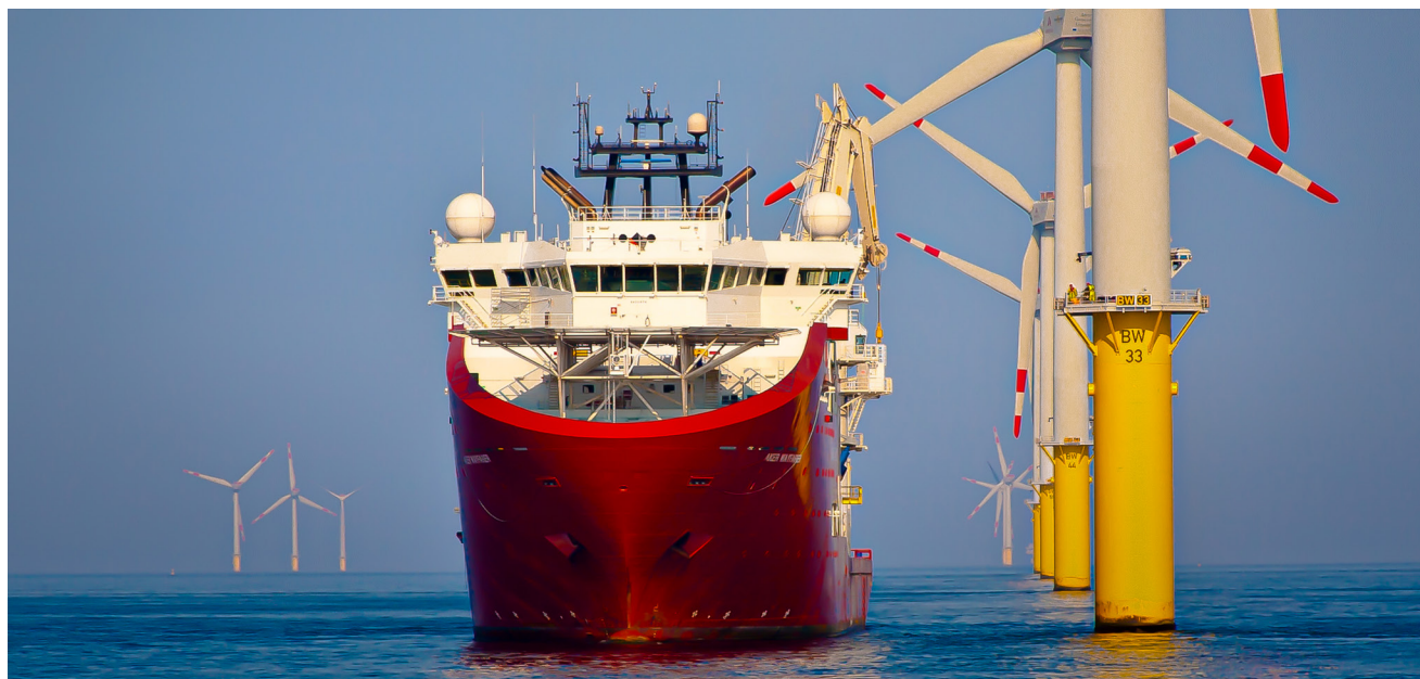
Figure 5. Service operation vessel that provides accommodations for workers during turbine service and repair work.
