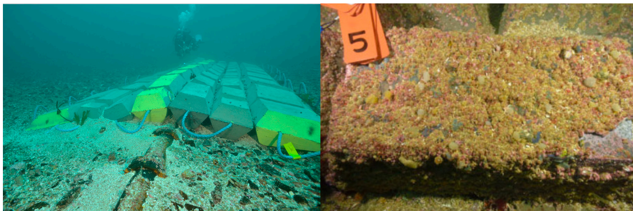
Figure 4. (Left) Newly installed concrete mattress over partially exposed subsea cable. (Right) Close-up image of concrete mattress that has been colonized by organisms after installation. Images from Taormina et al. (2020) .
