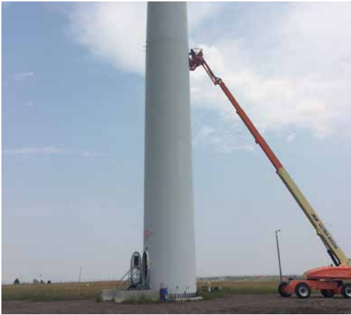
Figure 2. Light arrays being positioned below the sweep of wind turbine blades. Photo from Paul Cryan, USGS
