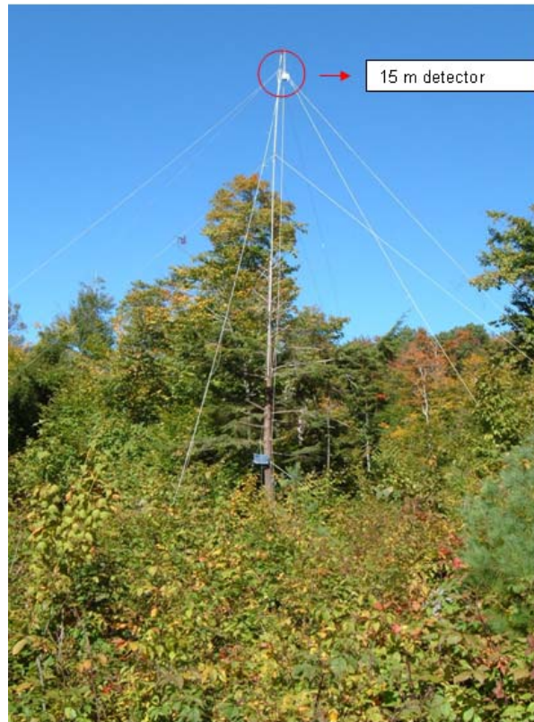
Photo 1: Fletcher Mountain North Portable Tower Detector
