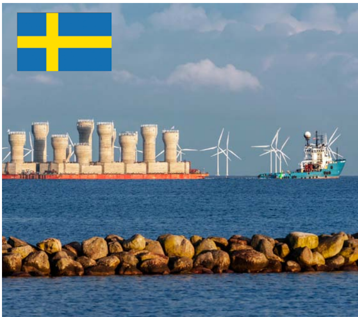
Milestone: Karehamn's gravity base foundations head out Photo: Eon
