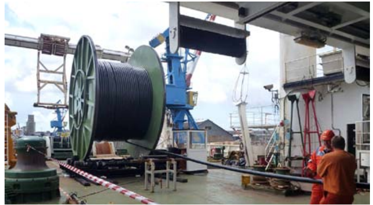
Le Croisic cable-laying: SEMREV is France's first grid-connected wave test site
