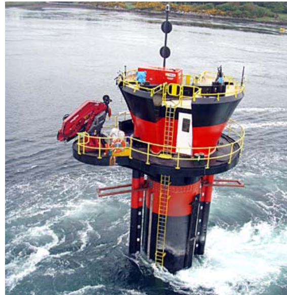
Developing strategy: Minas Basin Pulp & Power hopes to install a 3MW SeaGen-U unit, the fully submersible version of MCT's surface piercing tidal system
