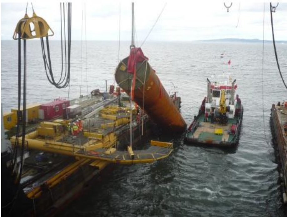
Svanen Piling Operations from http://www.bnoffshore.com/content/files/SITE4512/svanen.pdf
