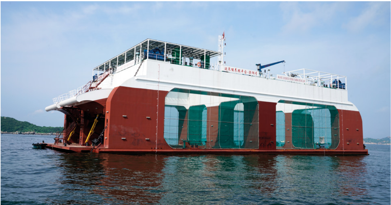
Penghu aquaculture platform (image courtesy of Guangzhou Institute of Energy Conversion Chinese Academy of Sciences).
