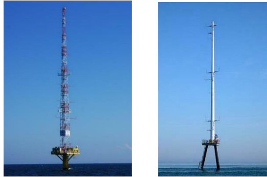
Figure 3.2 and 3.3: Lattice-mast meteorological tower with monopole foundation and monopole-mast meteorological tower (BOEM, 2015).
