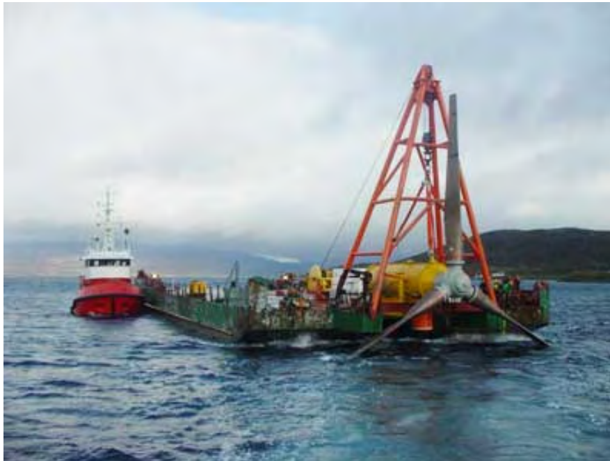
Figure 2.16 Hammerfest Strøm prototype turbine being installed at Kvalsundet [24]
