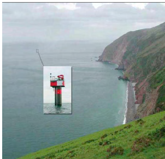
Figure 4.1 A photograph of Marine Current Turbine's Seaflow installation at Lynmouth, demonstrating the low visual impact of a single surface-piercing tidal stream device [62]
