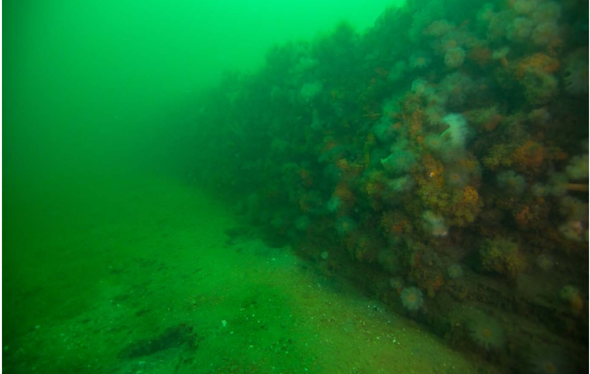
Figure 18. Wooden structure at Target 038.
