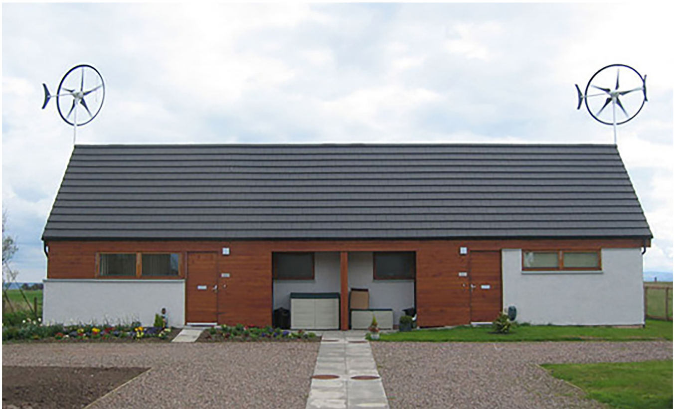
Fig. 9. Swift turbine installed on the roof of a small residential house [76].
