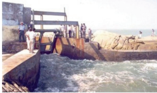
Fig. 2 Pendulum WEC with capacity of 30 kW at Dagan Island, Shandong Province
