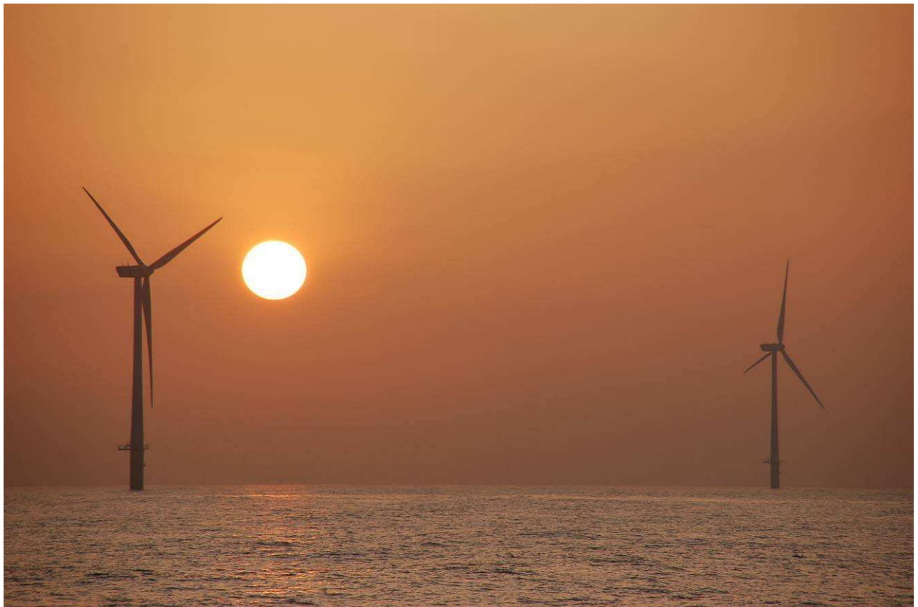
Photo 1. Two of the 36 wind turbines of the Offshore Wind farm near Egmond aan Zee (OWEZ) (Erwin Winter)
