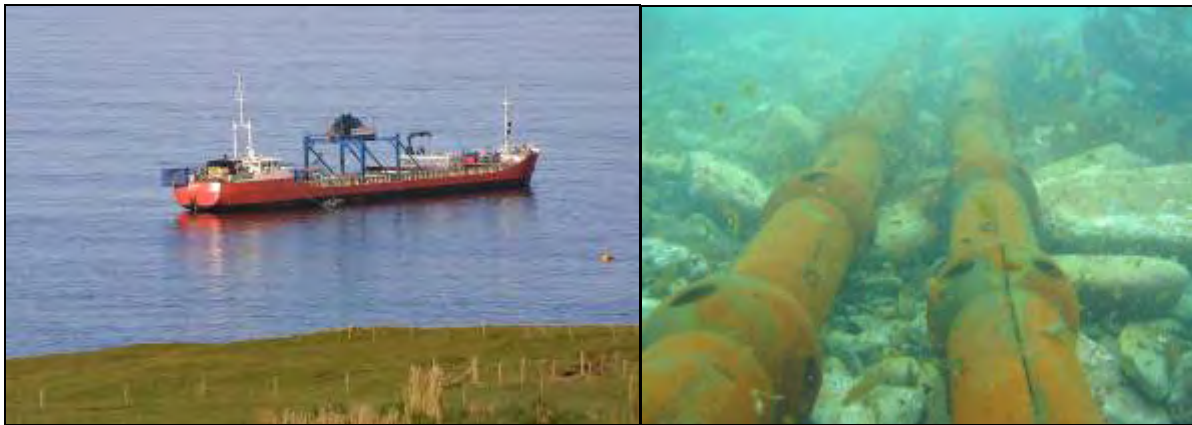
Figure 3.6 Cable ship Galathea (left) and ductile iron cable protection (right)
