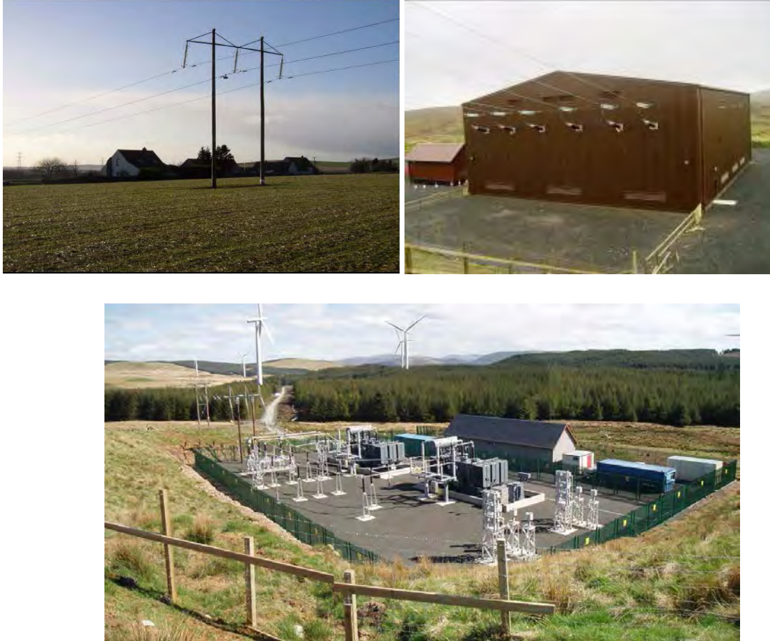
Figure 3.3 Example 132kV woodpole overhead lines (top left) and example 33/132kV enclosed substation (top right) and example 33/132kV outside substation (bottom)
