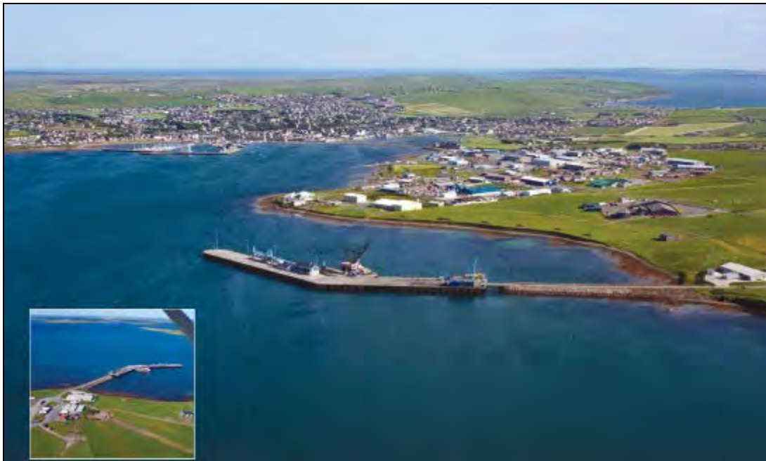
Figure 5.2 View of Hatston and Kirkwall Piers
