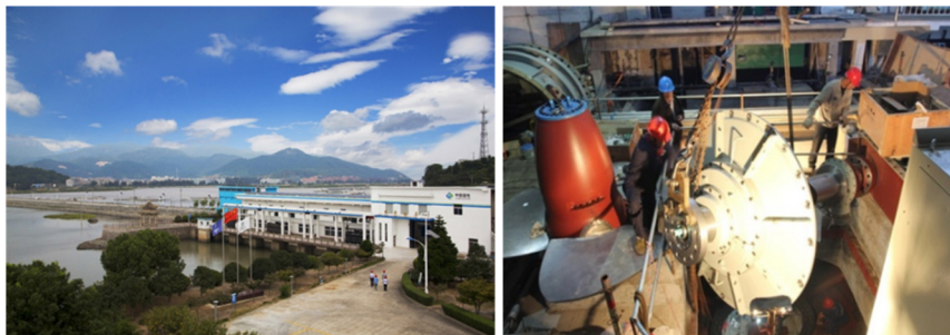
Figure 2. Jiangxia tidal power station and the turbine was being installed.
