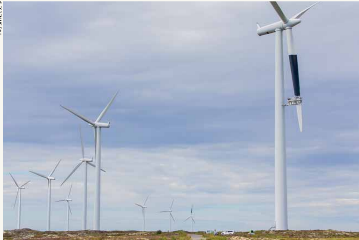
In Norway, at the Smøla wind power farm, experiments are currently being conducted on increasing the rotor blade visibility to birds by painting parts of the rotor blades black 194 .
