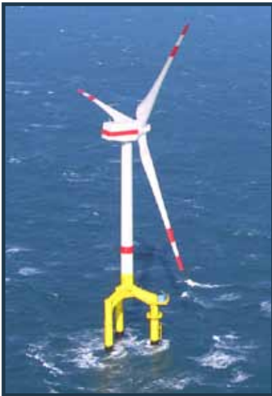
Figure 2a. Wind Turbine atop a Tripod Foundation at the Bard Offshore 1 Project. © BARD Group
