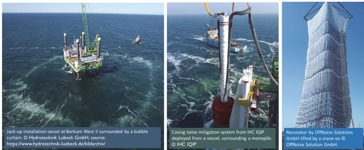
Figure 7. Examples of sound abatement systems including a bubble curtain (left), casing (middle), and resonator (right), figures adapted from Verfuss et al. 2019.
