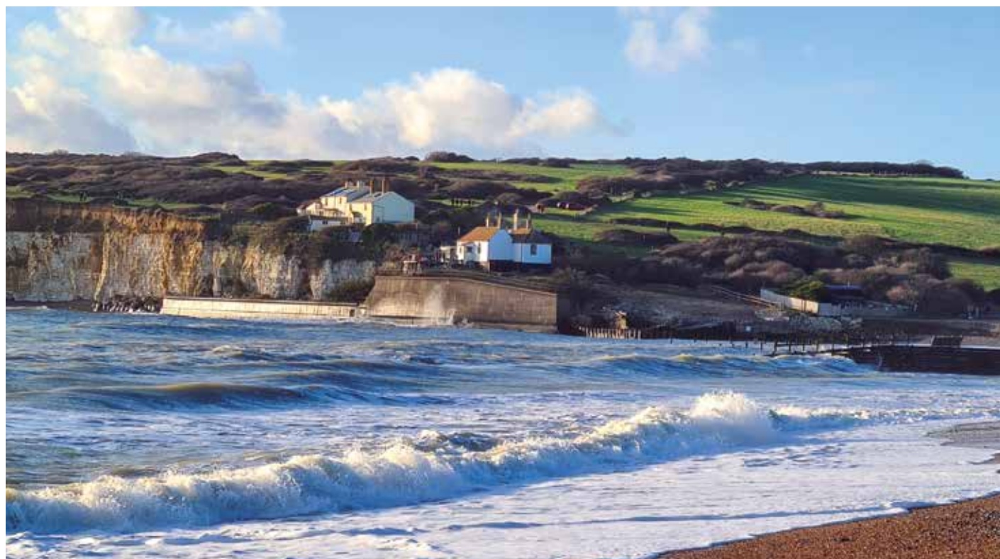
Houses at risk of falling into the sea due to eroding chalk cliffs at Birling Gap on the south coast of the UK.
