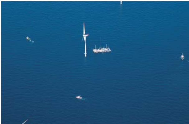
Photo 2. Horns Rev offshore wind farm under construction.
