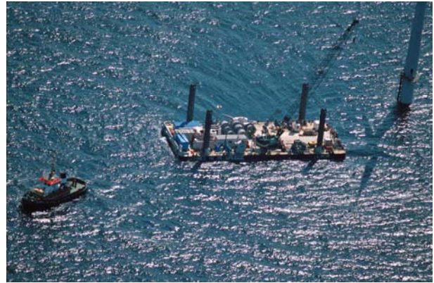
Photo 6. Horns Rev offshore wind farm under construction.
