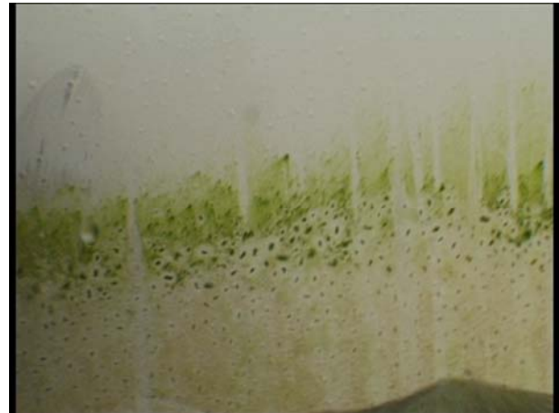
Photo 14. Larvae tubes of Telmatogeton japonicus (green dots inside white spots) in the splash zone at a monopile foundation.
