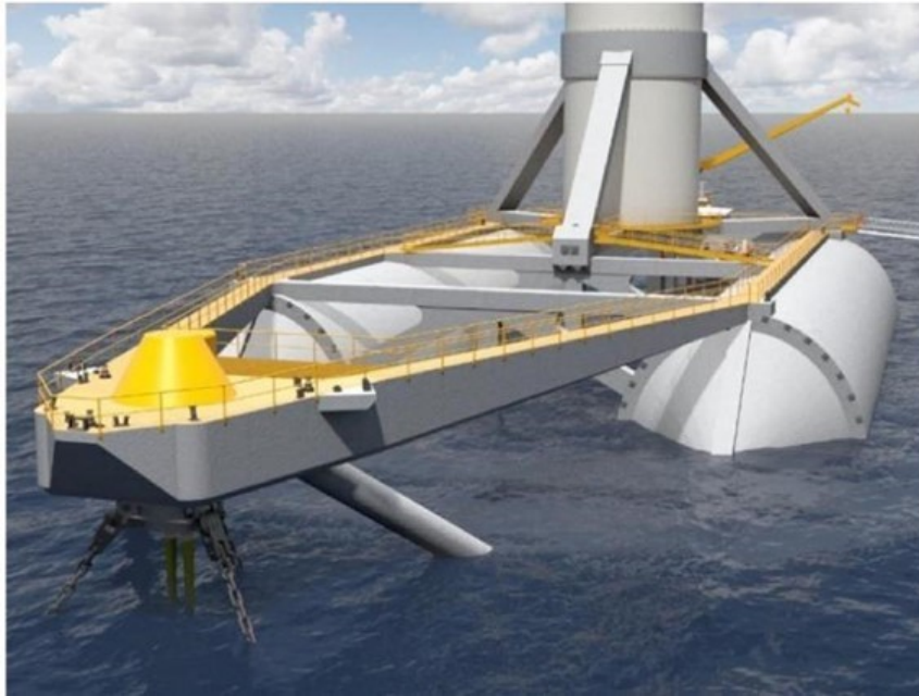
Figure 3-7. CADEMO Single Point Mooring (SPM) Connection
