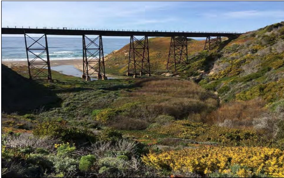
Figure 4-5. Mouth of Honda Creek and UPRR Bridge
