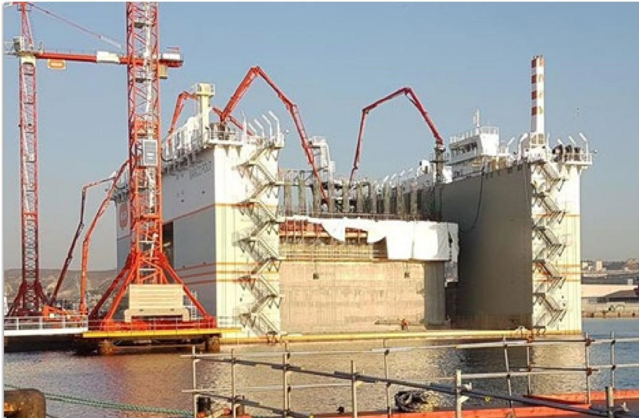
Figure 3-15. IDEOL Semi-Submersible Barge Construction Site Example
