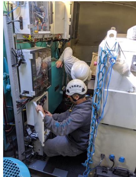
Figure 10. Natural Power and NREL staff up tower of the GE turbine while connecting the EchoSense system to the turbine network.
