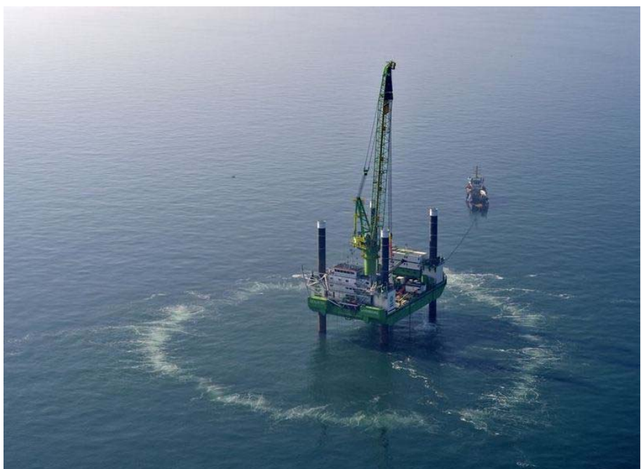
Figure 4.13. Example of active bubble curtain deployed around the jack-up platform used for pile driving. Air bubbles are visible in the surface as the white ring. The ship in the background is used for deployment and recovery of the hose system and contains the very large compressors needed to feed the bubble curtain with compressed air.
