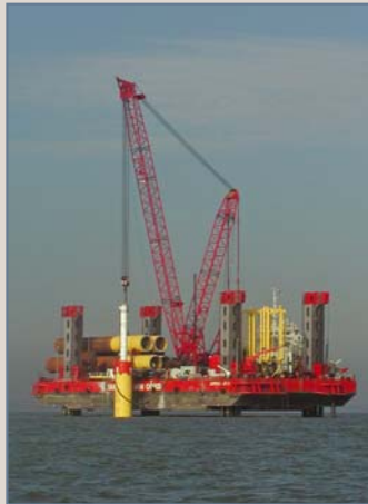
"Jumping Jack" pile driver
