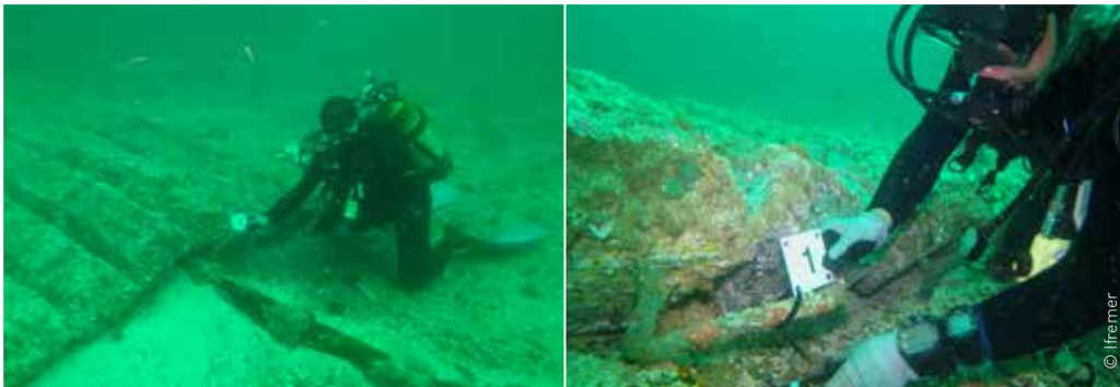
Fig. 51: Marking of the concrete mattresses inspected and the lobster shelters identified.
