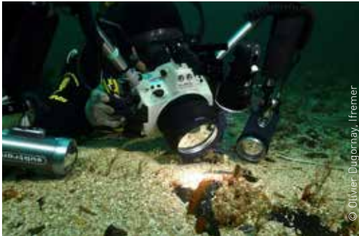
Fig. 50. Diver taking macrophotography of an invertebrate attached to the Paimpol-Bréhat test site power cable.
