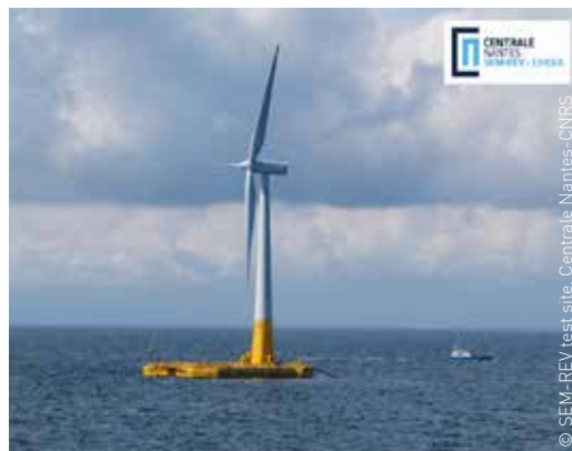
Fig. 49: Intervention at the SEM-REV test site.
