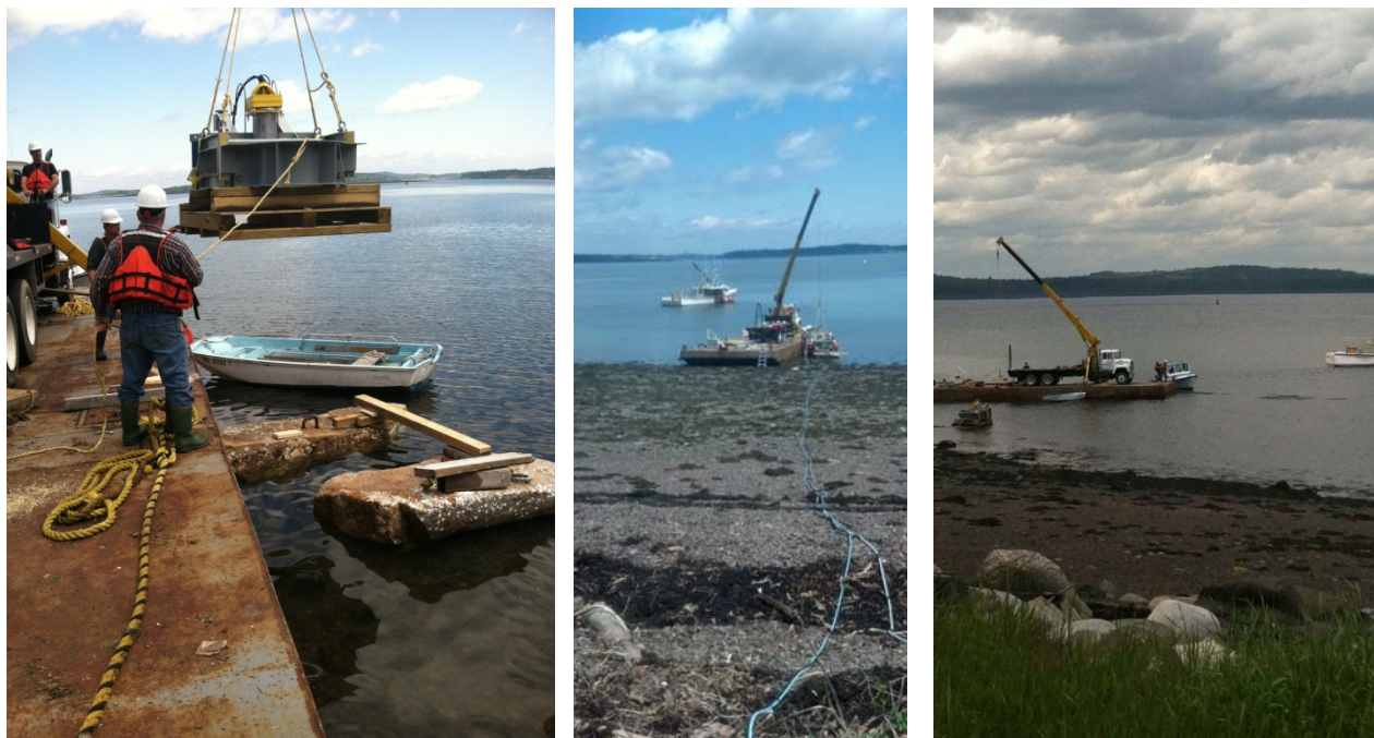
Figure 8: SDSN deployment procedure at low tide.
