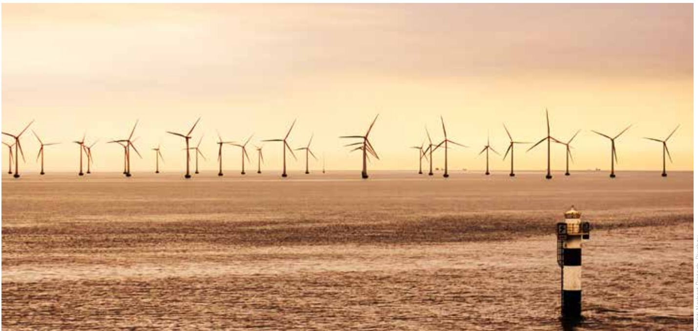
Wind turbines at sea.
