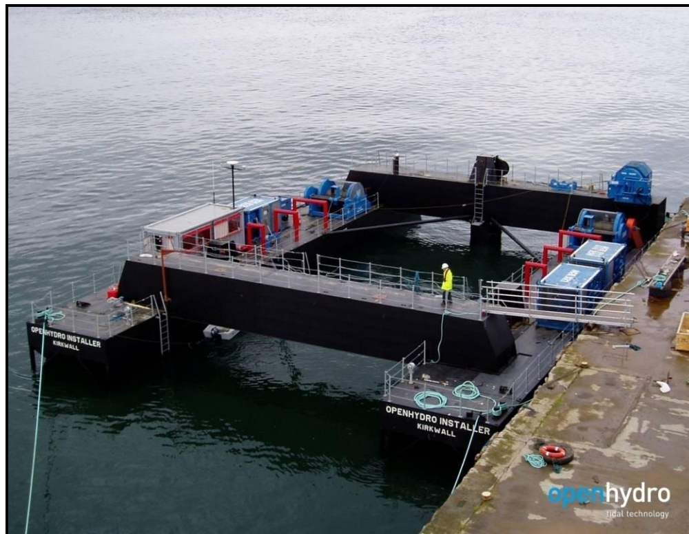
FIGURE 2-13 HEAVY LIFT OPENHYDRO TURBINE INSTALLATION BARGE
