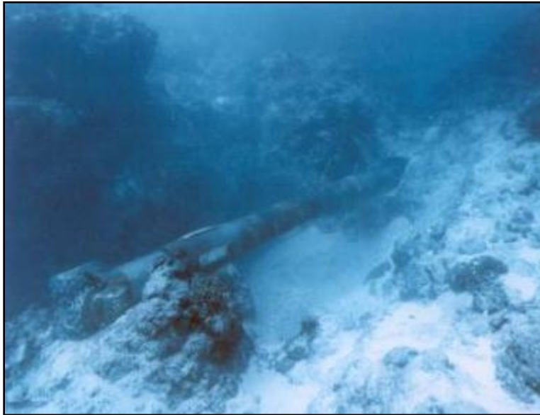
FIGURE 2-12 HDD DRILLING HEAD EXITING SEAFLOOR
