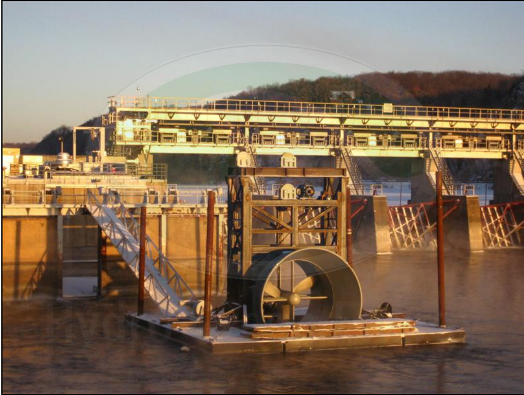
FIGURE 5-5 HYDRO GREEN ENERGY HYDROKINETIC TURBINE DEPLOYED IN THE TAILRACE OF THE U.S. ARMY CORPS OF ENGINEERS LOCK AND DAM NO. 2 ON THE MISSISSIPPI RIVER IN HASTINGS MINNESOTA (FERC NO. 4306)
