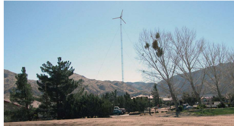
Bergey Excel 10, 10-kW wind turbine; Oak Hills, California. Photo by Karin Sinclair, NREL 14983
