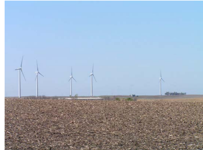
Junction Hill Top Wind Farm, Iowa. Five GE 1.6-megawatt (MW) turbines. Photo by Tom Wind, NREL 26494
