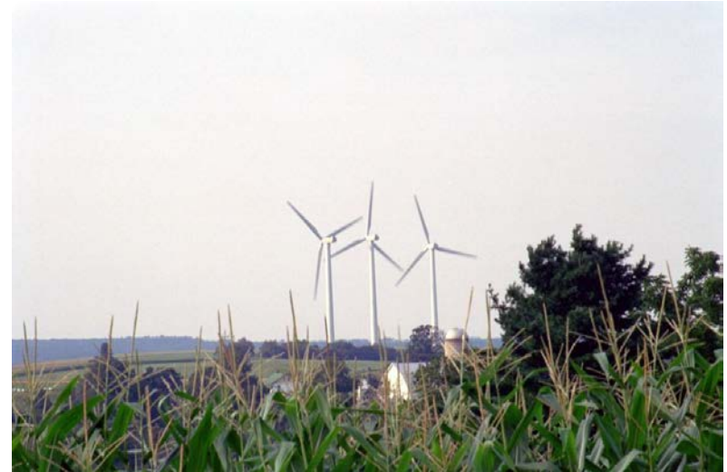
Eight Nordex N60, 1300-kW wind turbines; Garrett, Pennsylvania. Photo by Green Mountain Energy Company, NREL 09699
