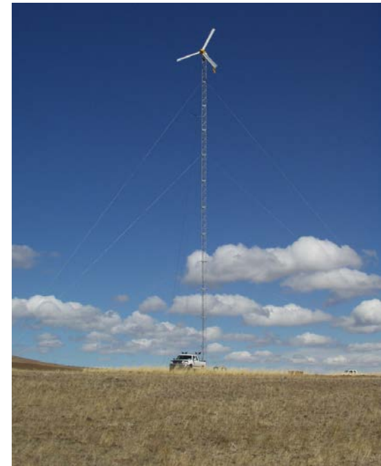
Bergey Excel 10, 10-kW turbine, Klickitat County, Washington Photo by Gwen Bassetti, NREL 26429
