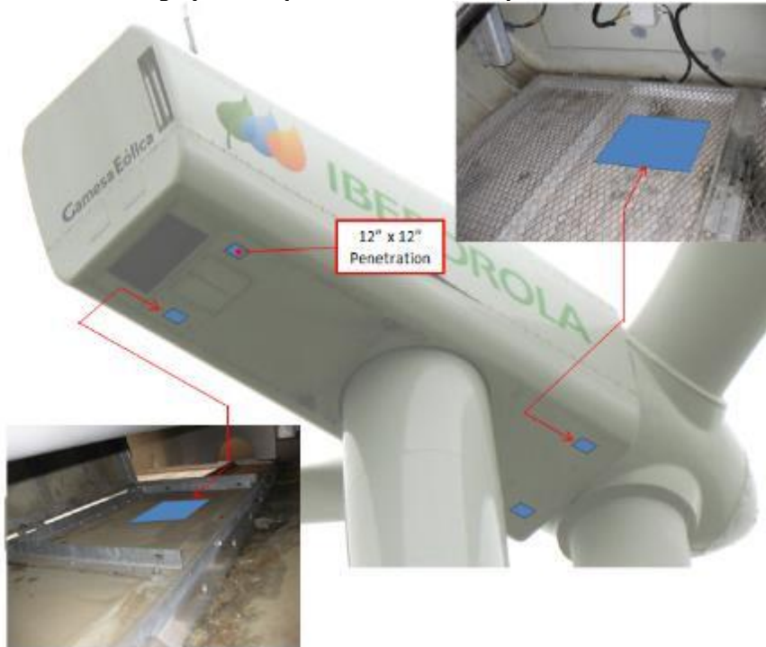
Figure 6. Placement options for UADs on the floor of the nacelle-viewed from the interior and exterior of the nacelle.
