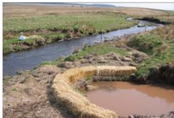
Sediment lagoons should always be situated away from watercourses, unless, as in this case, there are no alternatives. Better pre-construction planning should address this.
