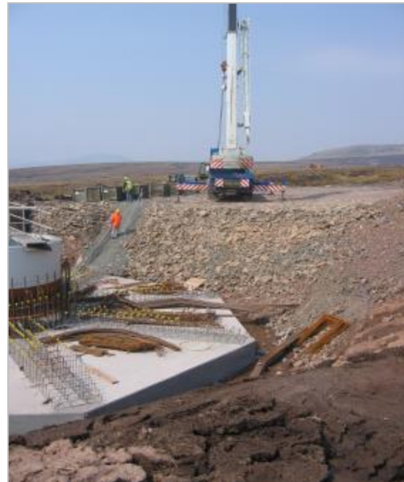
Turbine foundation under construction with adjoining crane pad.
