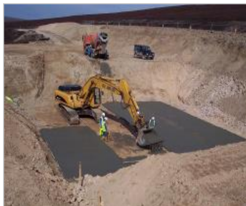
Preparation of turbine foundations
