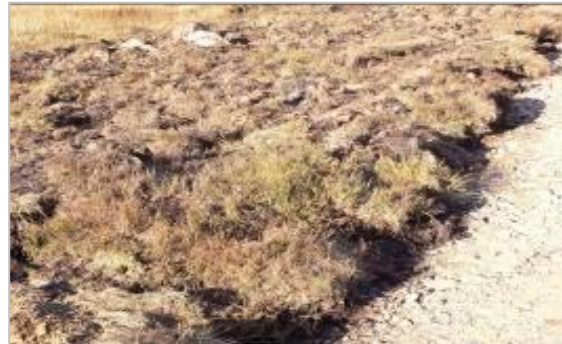
Reinstated turves at road verge provide optimal restoration. Careful supervision of works may be required to achieve this.
