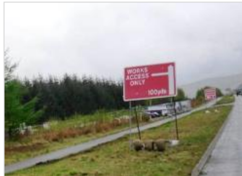
Use of road signs to inform other road users as well as drivers approaching site
