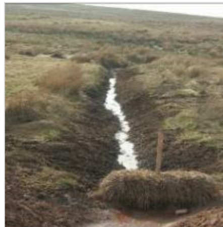
Straw bale 'pinned' in place
