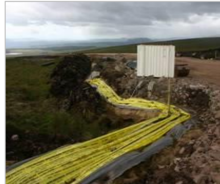
Cable trench adjacent to constructed road
