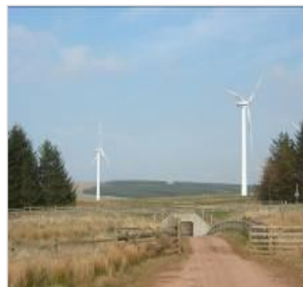
Maintaining access for a wide range of users will increase the benefits of the wind farm to the local community.
