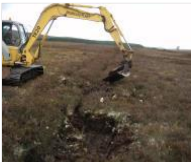
Peat dam construction
