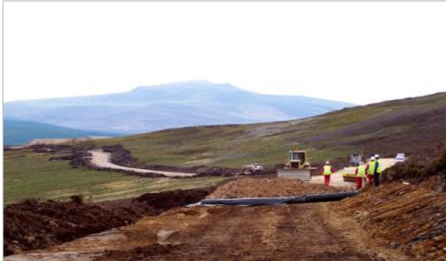
Construction of a cut road
