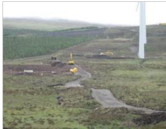
An example of good practice. Track edges have been reinstated with whole turves.
