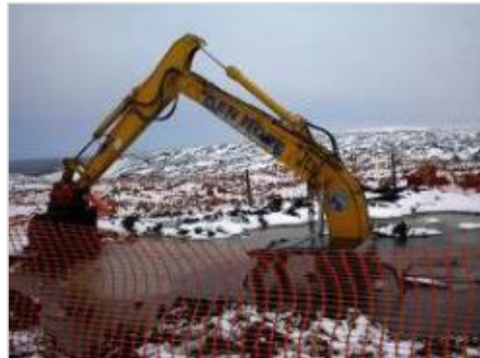
Winter conditions pose a significant challenge in all stages of construction
