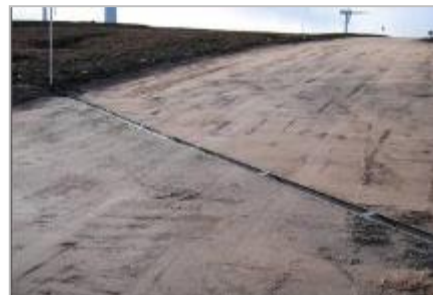
Cross-drain on access track
