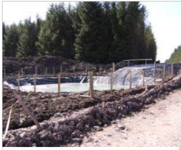
A well designed and located cement wash out bay can prevent bad practice elsewhere on site. A ticketing system to ensure it is used by all drivers has been shown to be useful.
