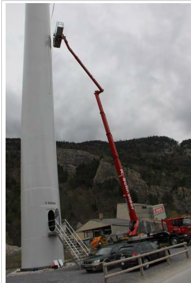
Installation at 31m height with man-lift
