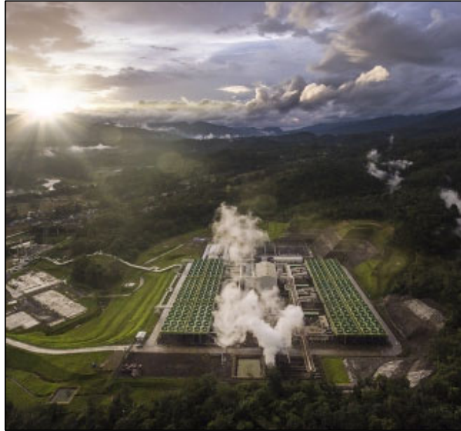
Figure 9.2: Sarulla Geothermal Plant, Indonesia
