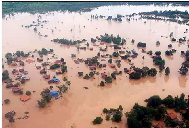
Figure 5.7: Downstream flooding following the collapse of Saddle Dam D in Lao PDR.
