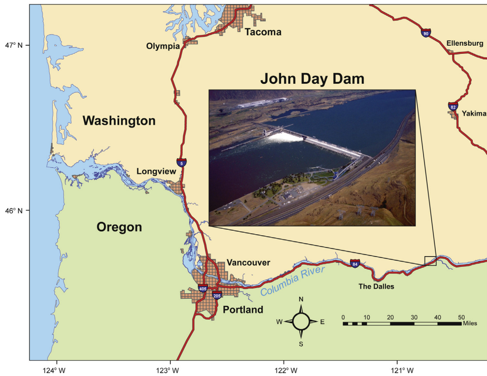
Fig. 6. John Day Dam on the Columbia River in the Pacific Northwest region of the USA.
