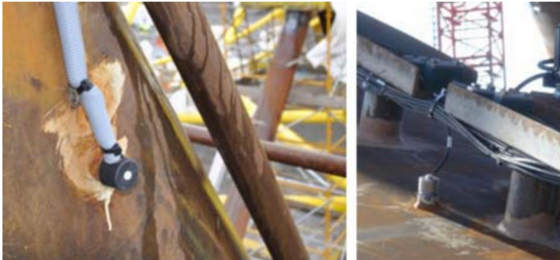
Fig. 6.1.2: Acceleration sensors on the foundation of the AV04 (left photo, source BSH) and on the lower brace of the foundation of the AV07 (right photo, source DEWI)
