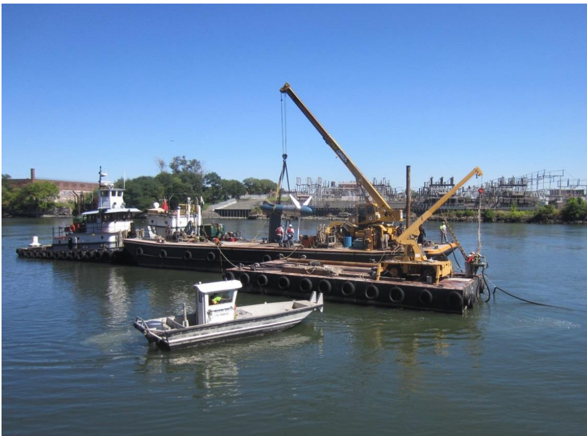
Figure 1-3. Gen5 KHPS turbine deployment with DIDSON (RAD) system being deployed (August 2012).
