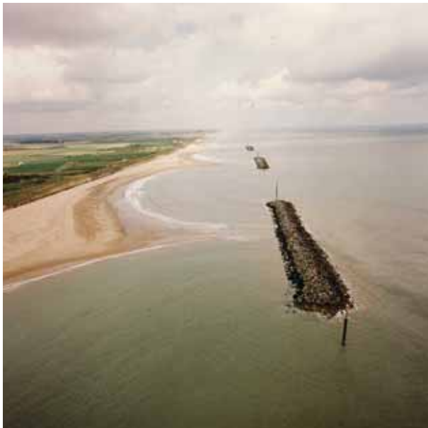
Figure 10: Part of the Happisburgh – Winterton coastal protection works (courtesy of Van Oord UK Ltd)
