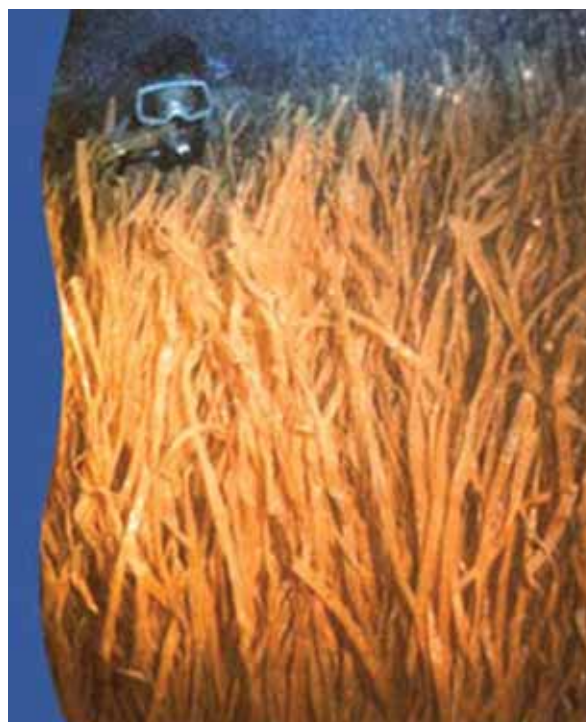
Figure 4: Turbine foundations: rock ballast (left) showing approximate scale and extent of optional rock-scour protection around turbines at North Hoyle (Ben Barton, formerly North Hoyle but now Crown Estate, June 2006, pers. comm.) and frond-mats (right) (reproduced courtesy of Seabed Scour Control Systems Ltd).
