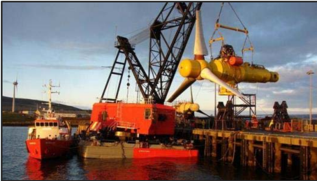
1 MW Alstom turbine mobilization (Orkney, UK)
