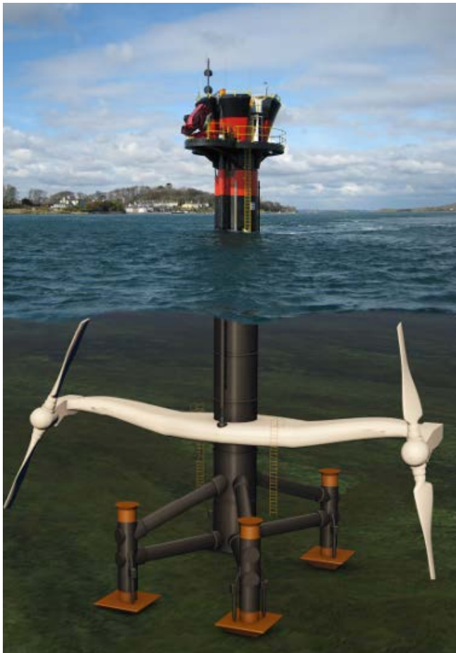
Figure 3. The SeaGen device: four-footed pin-pile foundation supporting the monopile (Royal Haskoning, 2011).
