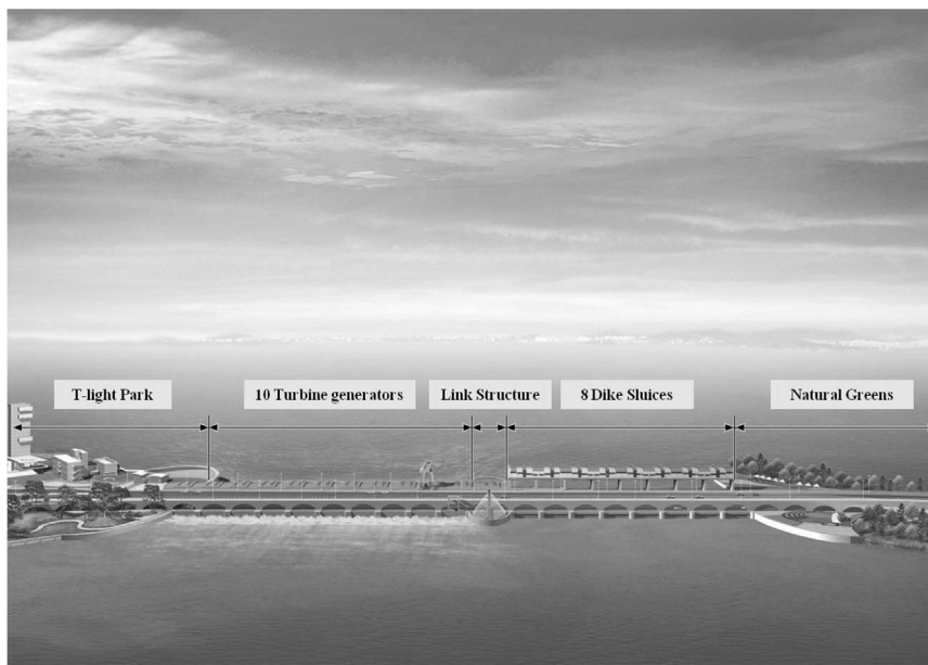
Fig. 6. Overview of the Shihwa tidal power plant.
