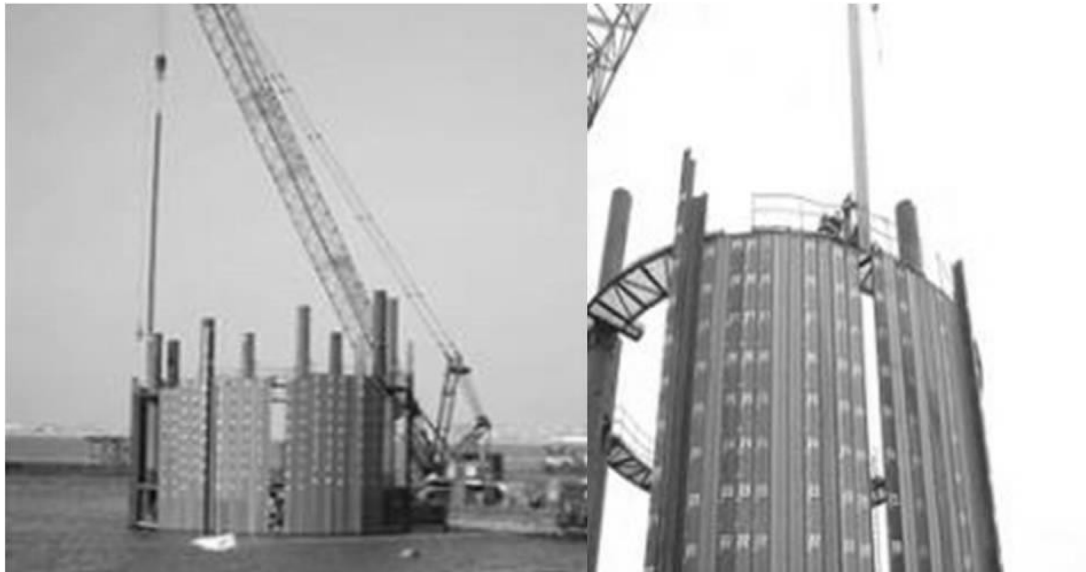
Fig. 12. Circular cell on site positioning and installation.
