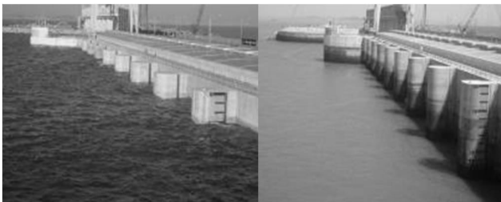
Fig. 7. Difference of the Shihwa lake water levels between rising tides and ebb tides.
