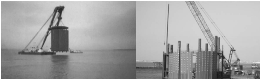
Fig. 14. Circular cell on land construction and marine transportation (left), on-site installation (right).
