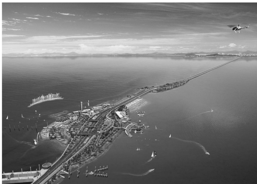
Fig. 1. The Shihwa tidal power plant.
