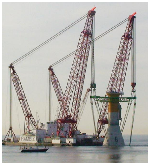
Figure 2.17 A typical gravity base caisson foundation for shallow depth (left © https://www.wind-energy-the-facts.org/offshore-support-structures.html ) A gravity foundation being installed at Thornton Bank by the heavy lift vessel Rambiz (right, source & © LUC VAN BRAEKEL)
