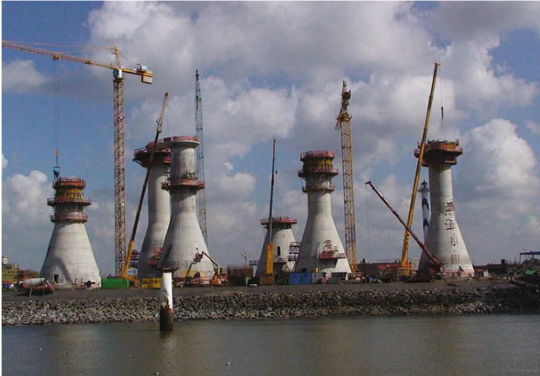
Figure 2.3 Gravity foundations under construction for Thornton Bank (source: LUC VAN BRAEKEL).
