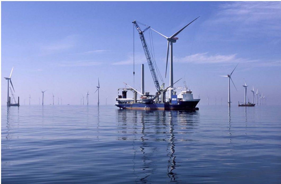
Construction of an offshore wind farm – Horns rev 2
