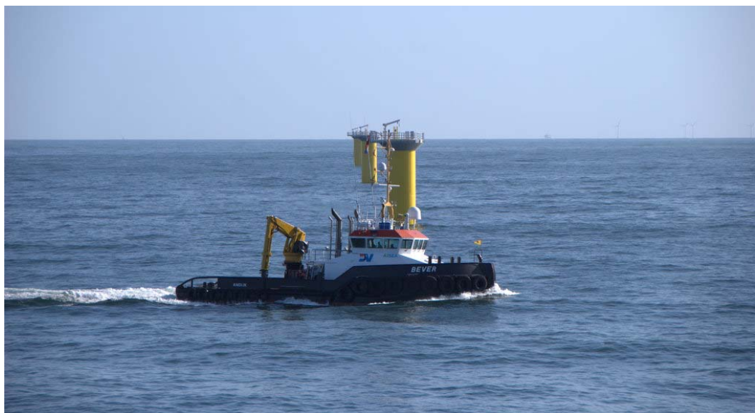
Installation of monopiles at Horns Rev 2
