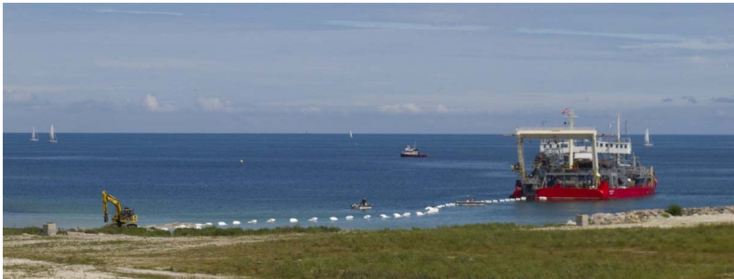
Cable laying vessel near shore
