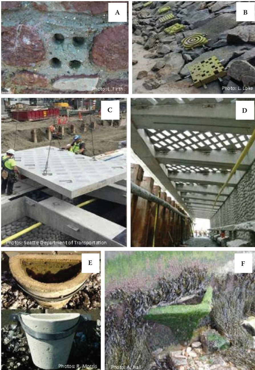
Figure 11 Variety of different ecological engineering techniques that can be incorporated onto seawalls. (A) Pits created by manipulating the concrete between bricks on a seawall, Shaldon, United Kingdom (Firth et al. 2014b). (B) Precast habitat enhancement plates/tiles with different levels of complexity affixed to a seawall in Pulau Hantu, Singapore (Loke et al. 2014, 2015). (C, D) Large-scale precast fascia fronting urban seawalls in Seattle, Washington, USA (Toft et al. 2010, 2013). (E) Modified precast concrete flowerpots affixed to seawalls in Sydney, Australia (Browne & Chapman 2011, 2014, Morris 2016). (F) Precast concrete Vertipool affixed to seawall on the Isle of Wight, United Kingdom ( http://www.ecclestonegeorge.co.uk ).
