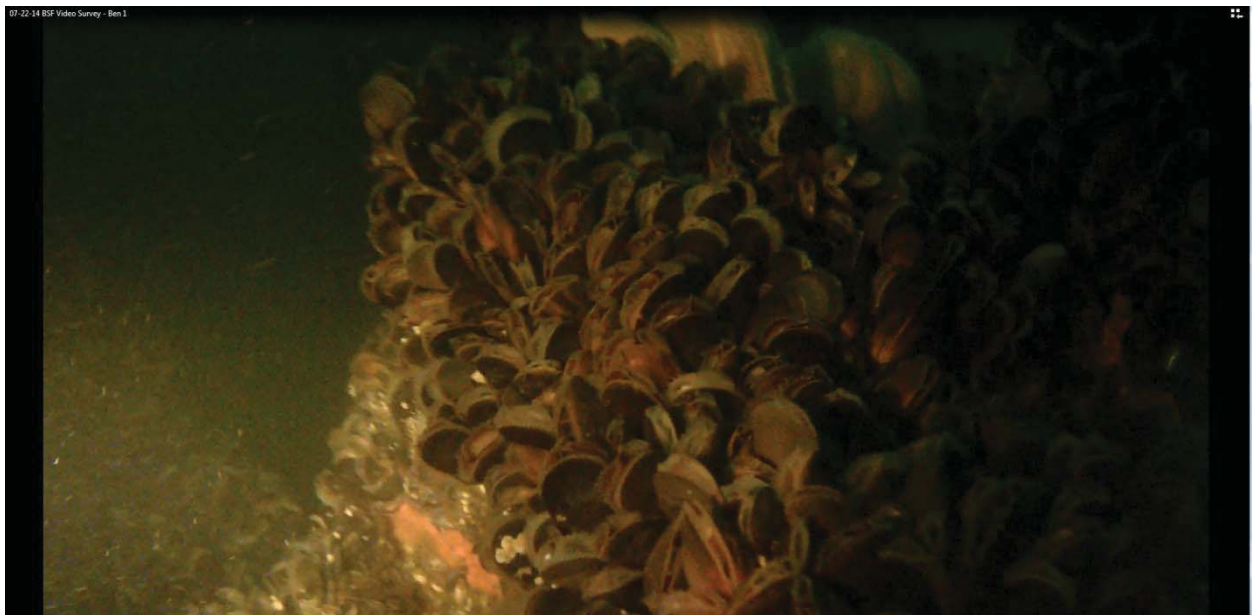
Figure 8. Blue mussels on steel pile (center) and bottom support frame (lower left)
