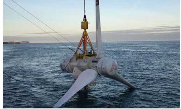
Deployment of SIMEC Atlantis' AR1500 turbine at MeyGen (© SIMEC Atlantis)
