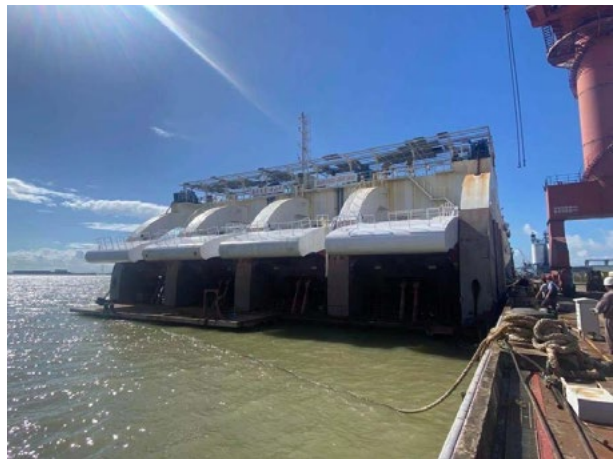
“Zhoushan” under maintenance
