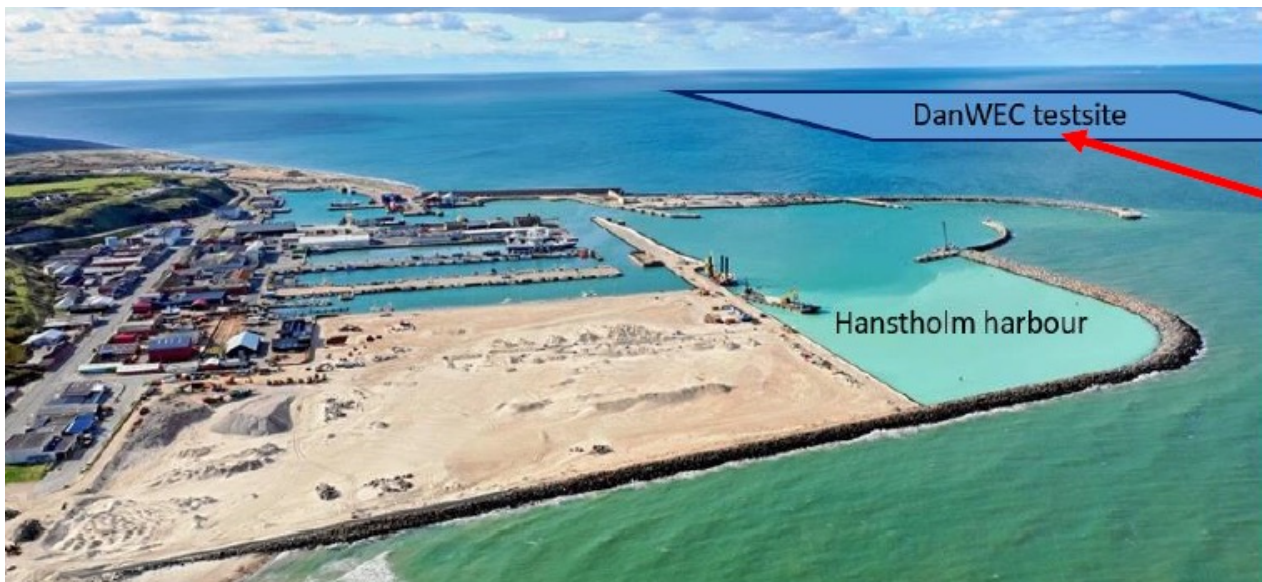
Picture of the Hanstholm harbour and the location of the DanWEC test site
