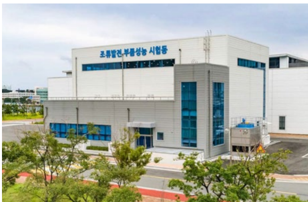
Tidal energy component experiment building and actuators for testing (Courtesy: KIOST)
