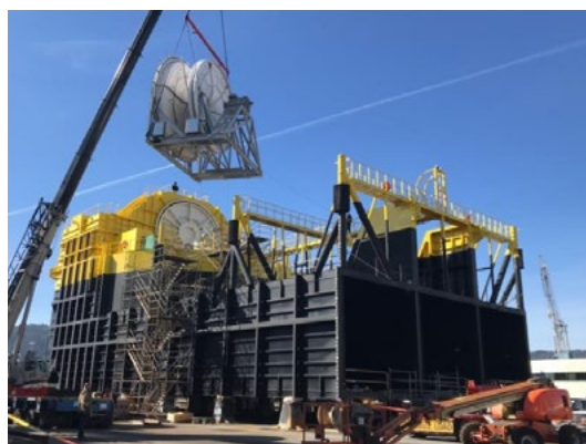
OE Bouy during construction in Oregon
