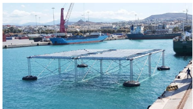
Current build-out of SINN Power's SOcean hybrid platform at the port of Heraklion
