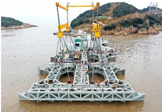
Platform being installed
