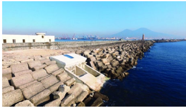
Breakwater equipped with the OBREC prototype in the Naples harbour
