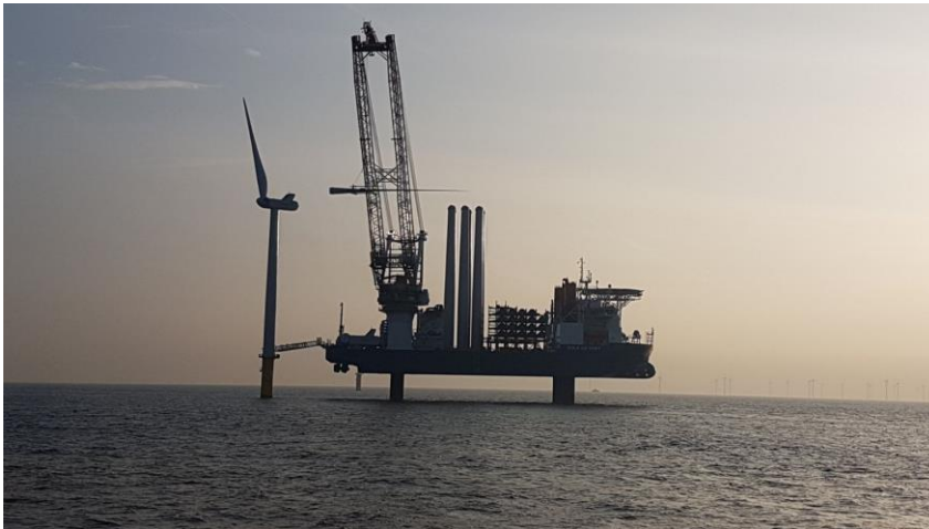
Figure 4: Installation of WTG
