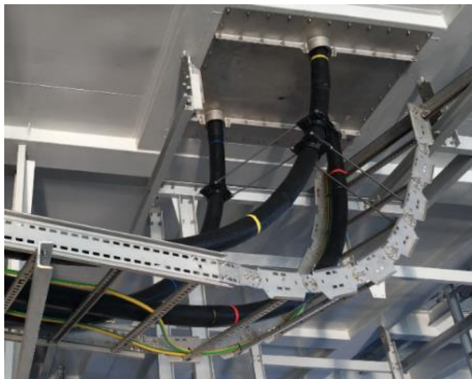
Figure 5: Fixation 220 kV export cable
