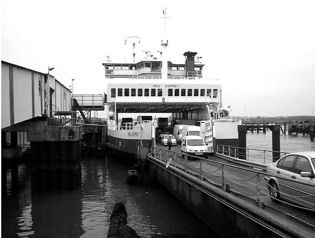
Fig. 1. Photograph taken from quayside with ferry docked at terminal, and vehicles disembarking along linkspan. Structure on left of photograph is covered walkway for pedestrian passengers, and the dolphin on which it rests can be seen.
