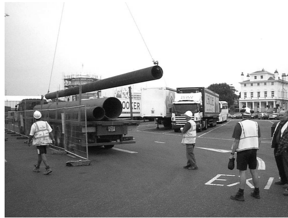
Fig. 8. Photograph of pile tubes being unloaded from lorry.
