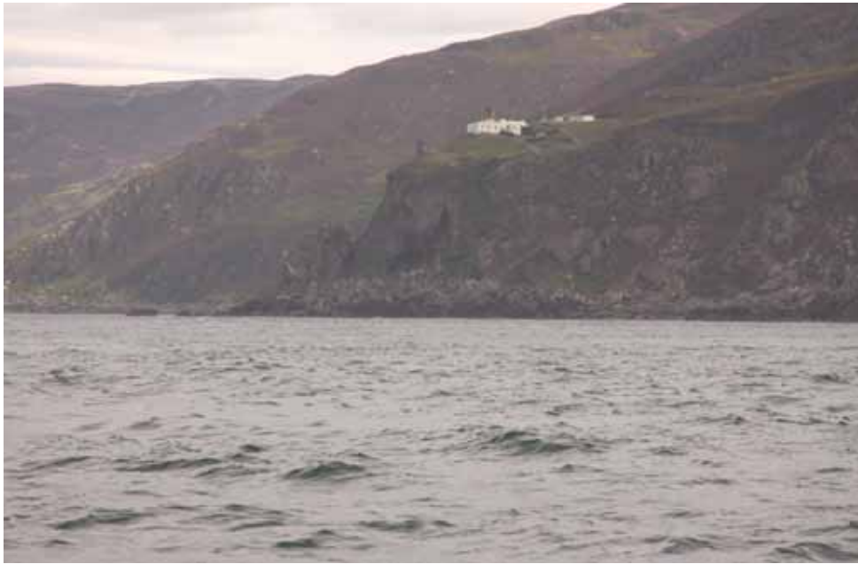
Figure 14.3 – Typical view of the lighthouse from the sea
