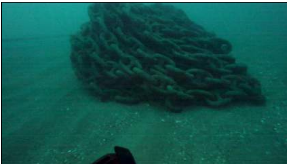
Figure 30. Ripple marks close to one of the chain weights of mooring leg 1.
