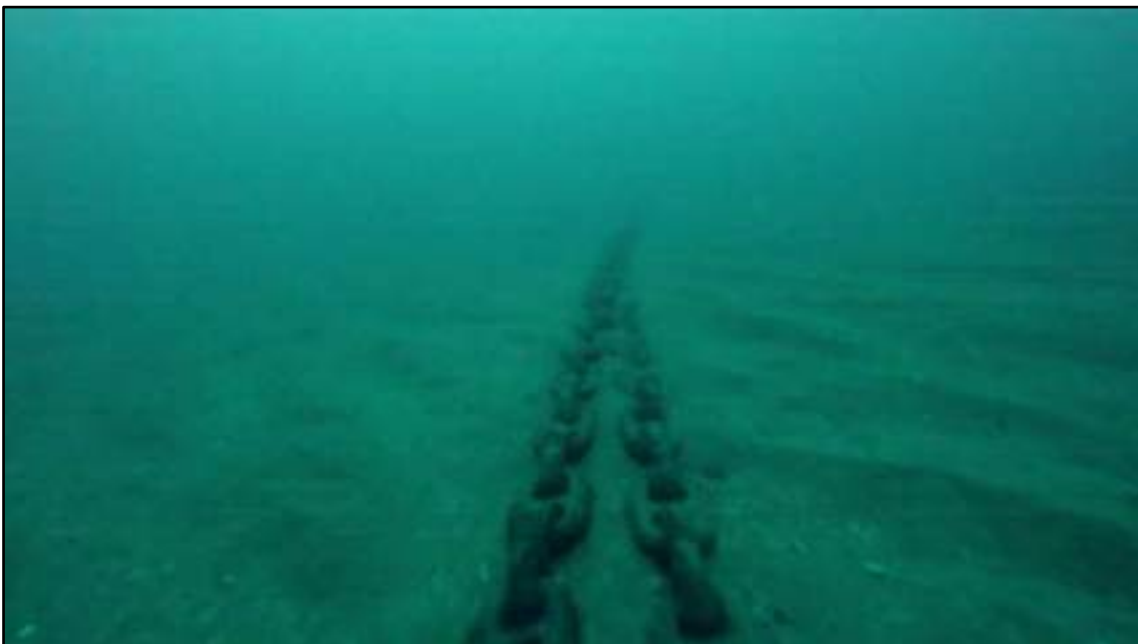
Figure 36. Lower catenary of the mooring leg 6.
