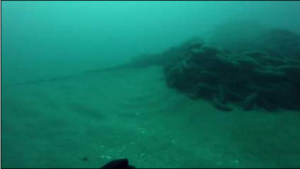
Figure 37. Sand accumulation in the western side of the chain weight CW5a.
